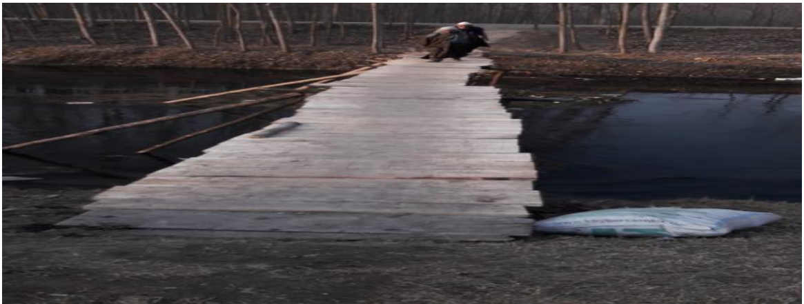
Bridge between Darhpora Korag Domarg and Wakoora Block
