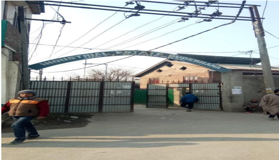
Figure 1: Industrial Estate Ganderbal within locality
