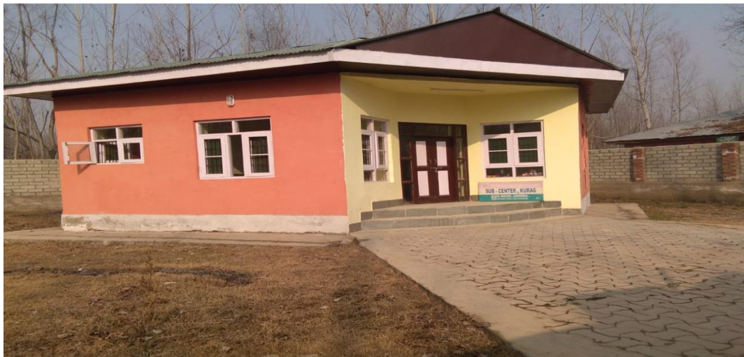
Figure 11: Newly constructed sub-center in village Korag Domarg
